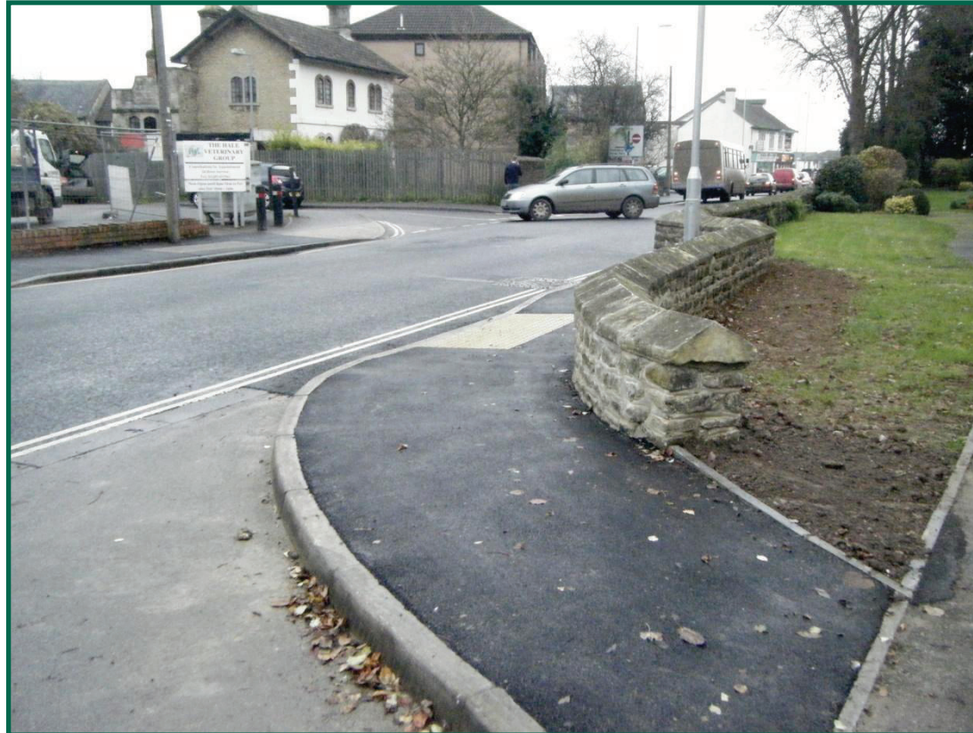
Langley Road - Footway Link & crossing point AFTER
